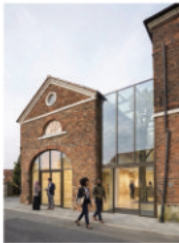
Reinstated arched entrance and vertical circulation lift
